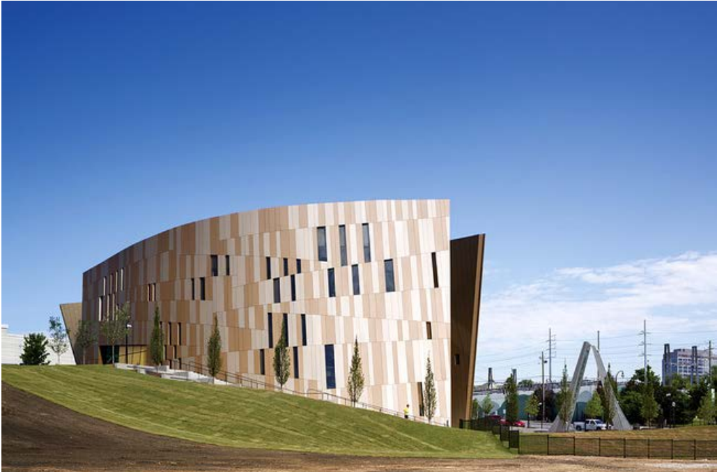
Photo © Albert Vecerka/Esto Designed for LEED Gold certification, the Center is set into a hillside facing Atlanta's Pemberton Place, a pedestrian park. SLIDE SHOW
